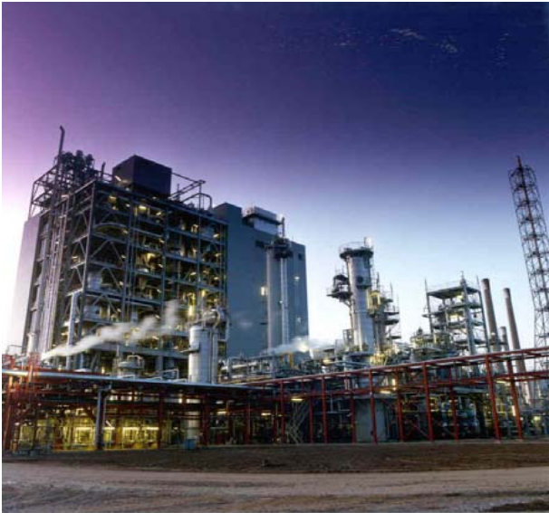
Nuon's clean coal plant in Buggenum
